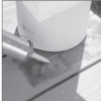
4. Apply construction adhesive\* to top and bottom surfaces of column.
