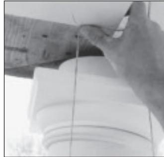
5. Put assembly in place and plumb. Make sure load is centered over column shaft and evenly distributed around the bearing surface.
