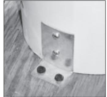
6. Mark and drill holes in floor and column shaft for corner/ angle brackets (not included). (HB&G column installation kit available #17040)
