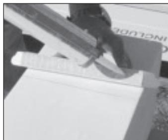
9. Mark location for supplied neck molding. Measure and cut neck molding to a 45° angle. Apply construction adhesive\* and put neck mold in place.
