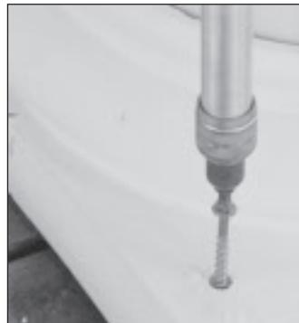
8. Apply construction adhesive\* to bottom of base and nail or screw to floor.
