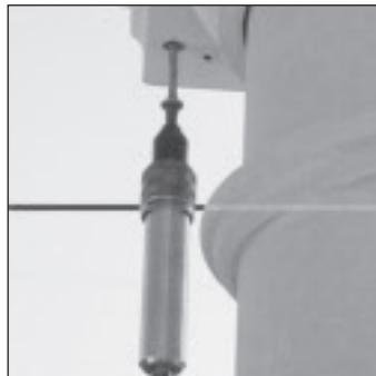
7. Apply construction adhesive\* to top of cap, press against structure, and screw or nail into place.
